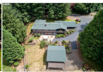
Exterior - NE Facing
