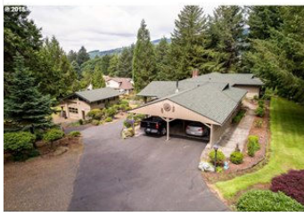
Exterior - West Facing
